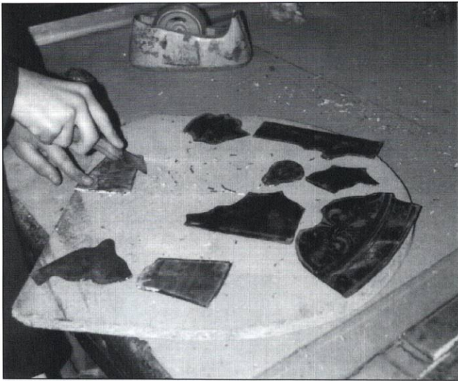
The perished lead was stripped away and each piece of glass cleaned.
