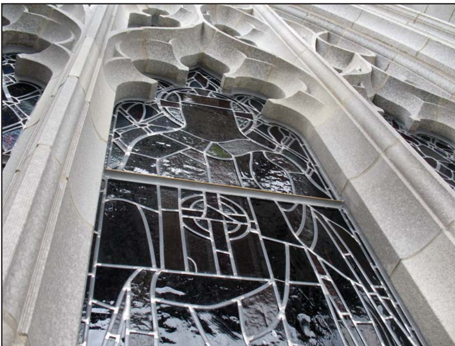
A lancet window with a new perimeter sealant joint.
