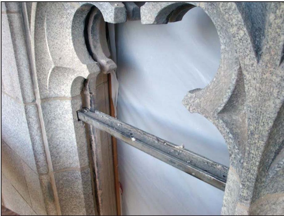
A stainless steel cross bar provides additional structural support.
