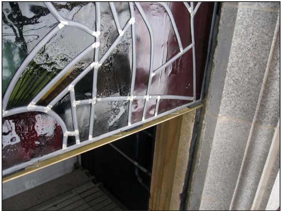
Exterior detail of new tee bar installation.
